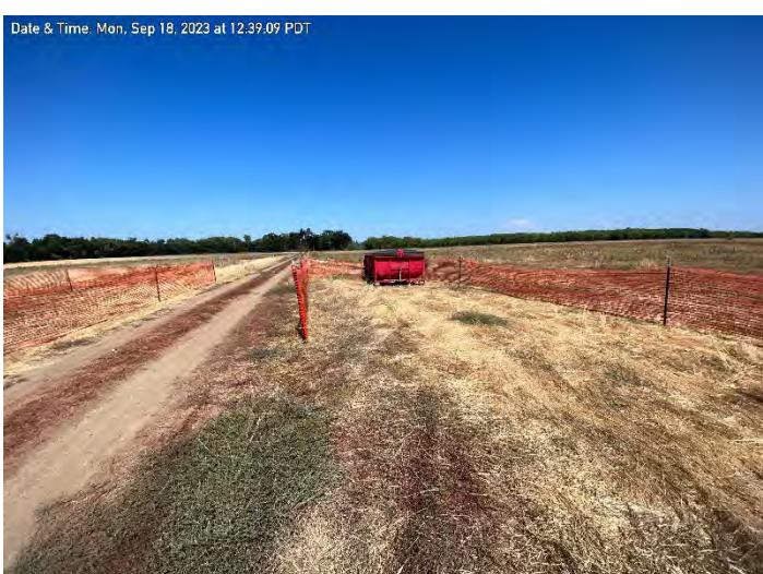
Photo 5: Construction fencing delineating work and staging areas, looking northeast. Note soil roll off bin.
