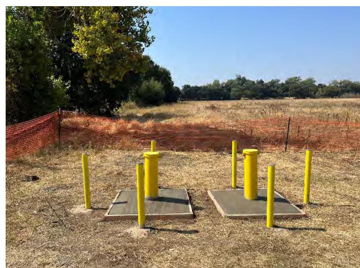
Photo 12: Completed wells GS-S (right) and GS-M (left), looking west.
