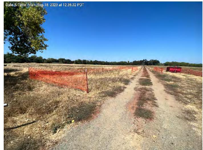
Photo 4: Construction fencing delineating work and staging areas, looking northwest.
