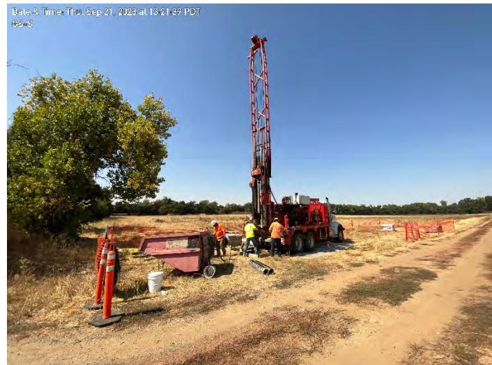
Photo 8: Hollow stem auger rig advancing well GS-S, looking northwest.
