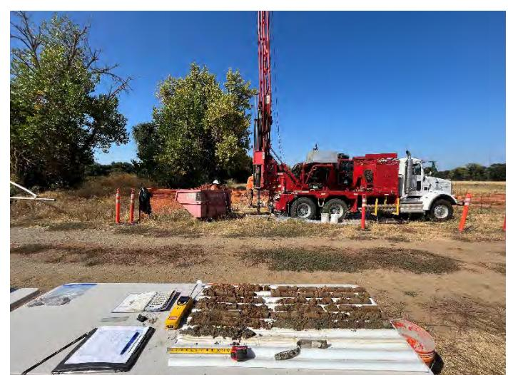
Photo 6: Hollow stem auger rig advancing well GS-M, looking west.
